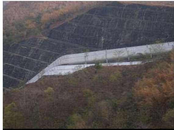
Water flow from the penstock
