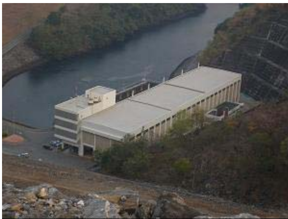
The Hydro-power Station
